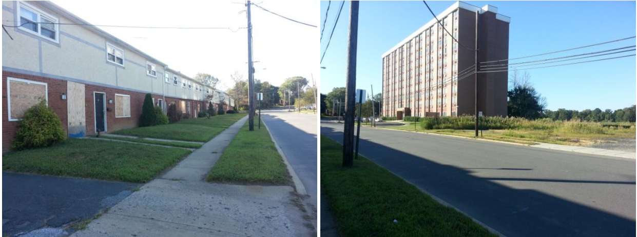
Figure 3: The 15 unit townhouse development at 45 Beers Street (left) remains vacant after taking 6 feet of water from Sandy's surge. The ten story Keyport Legion Apartments at 30 Beers Street across the street had 4 feet on the ground floor. The tidal marsh from the Lappatong Creek is visible directly behind the highrise building.
