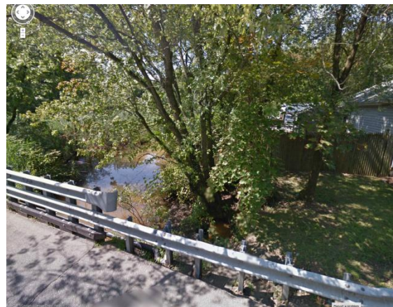
Figure 15: Google Street view of bridge at Green Grove Avenue
