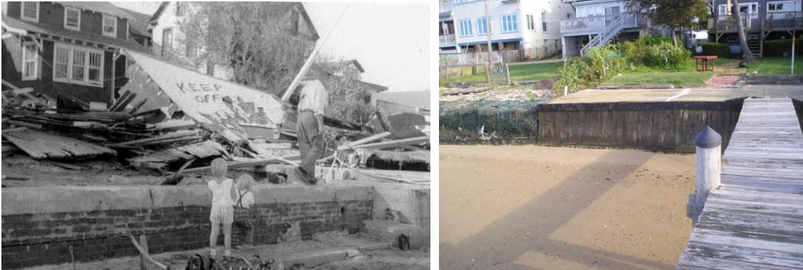
Figure 7 (Left): Bulkhead photo at 51-53 First Street after Hurricane Belle destroyed the garage at 55 First Street. The bulkhead at this time (9/1976) was ~ 2.5 feet in height above the beach. (Right): Bulkhead photo at 51 First Street after the 1992 December Northeaster, which pushed water up to the basement door sill (elevation 11.5 ft). The bulkhead at this time (12/1992) was ~ 5 feet in height above the beach. Courtesy of Michael Lane, Keyport, NJ
