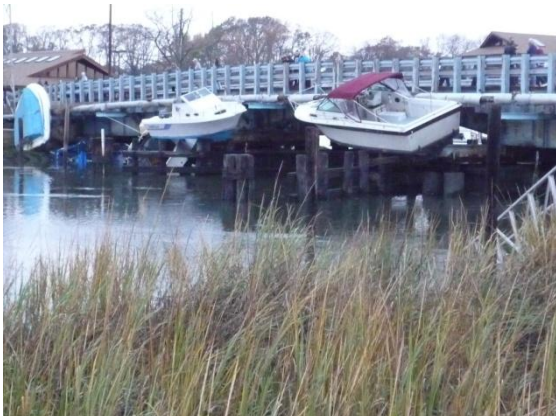
Figure 5: Boats are left hanging from the bridge at the Lappatong Creek after Sandy's surge subsided. The marine businesses, such as the Keyport Marine Basin and Pederson's Marina suffered heavy damage to facilities and loss of boats from 6 to 10 feet of floodwater ( image from bing.com )
